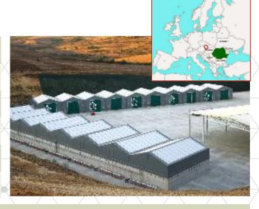
WITH THE TURTLE™ BIOCELLS SYSTEM, ENTSORGA ENABLED THE COMMUNITY OF GALDA DE JOS AND THE PROVINCE OF ALBA JULIA TO MANAGE MORE EFFICIENTLY MUNICIPAL SOLID WASTE BY PREPROCESSING MSW PRIOR TO LANDFILLING. THIS SUBSTANTIALLY IMPROVED THE ENVIRONMENTAL IMPACT OF THE DISPOSAL SYSTEM BY REDUCING VOLUMES LANDFILLED, LEACHATE PRODUCED AND RELEVANT GREENHOUSE GASES EMISSIONS.
