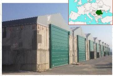
BY PROVIDING A **BIOCELLE TURTLE™ SYSTEM**, ENTSORGA IS HELPING THE COMMUNITY IN THE MARAMURES DISTRICT **TO STABILIZE THE UNSORTED SOLID WASTE**, REDUCE ITS VOLUME AND PRODUCE A **COMPOST LIKE OUTPUT** SUITABLE FOR A SAFER LOWER IMPACT DISPOSAL.
